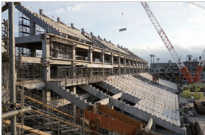
A stadium under construction
