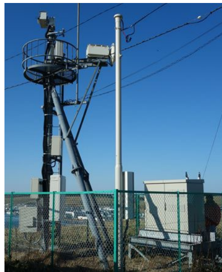
DMFC in use as live camera uninterruptible power supply
