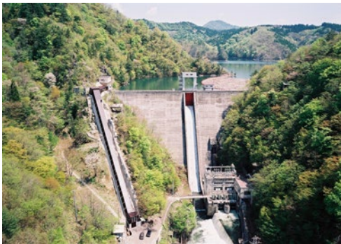
The Komatagawa No. 4 Hydroelectric Power Plant, completed in 1953, and Moriyoshi dam
