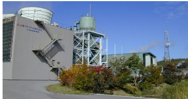
The Onuma Geothermal Power Plant completed in 1974, Japan's third geothermal power plant
