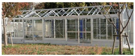
MKK's photobioreactor features an original reactor frame with seismic isolation structure (patent pending) to minimize damage by vibration as well as flying objects as countermeasures against large earthquakes and typhoons.
