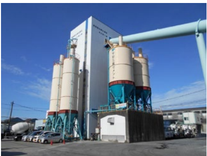
A plant producing ready-mixed concrete.
