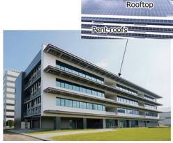
SUSTIE® exterior. Equipped with solar panels only on the rooftop and pent roofs, the test facility shows that ZEB can be deployed even in urban areas with restricted site areas.
