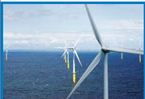
North Hoyle Wind Farm, located off the North Wales coast and capable of powering 40,000 homes, was partly financed by Bank of Tokyo-Mitsubishi UFJ
