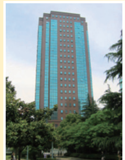
The AEtina Tower in Shanghai, which houses the headquarters of Mitsubishi Rayon (Shanghai) Co., Ltd., is strategically located near the web of expressways between the Hong Qiao Airport and the suburbs—an excellent spot for sales activities...
