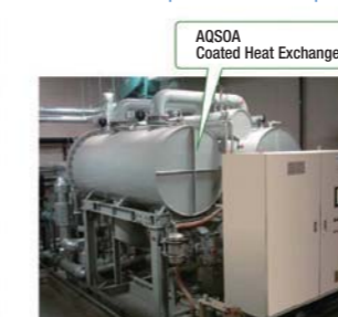
AQSOA Adsorption Heat Pump
