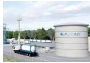
Brunei Hydrogen Production & Hydrogenation Plant
