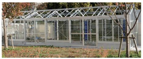
MKK's photobioreactor features an original reactor frame with seismic isolation structure (patent pending) to minimize damage by vibration as well as flying objects as countermeasures against large earthquakes and typhoons.
