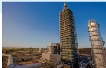
World's largest post-combustion CO 2 capture system (Houston, Texas, USA)
