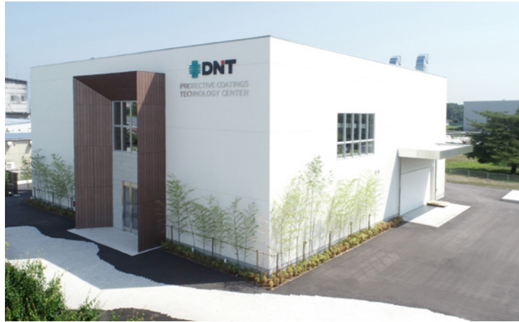
Protective Coatings Technology Center exterior
